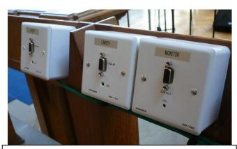
All visual connectivity utilises Kramer Twisted-pair (cat5e) distribution. Three active Kramer WP-110/120 plates on the platform are installed for laptop and roaming camera input with a monitor output for a TFT/LCD display.
