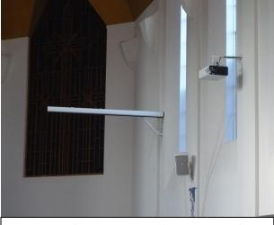
Sanyo 6500 lumen projector and custom screen that folds back discreetly against the wall when not in use
